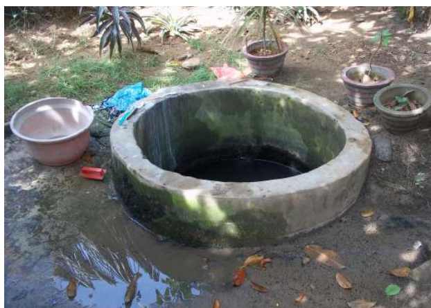
Figure 14: Dug wells with poorly constructed wall.
